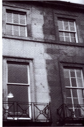
Figure 8.32 Other situations, where the cleaning material is clearly inappropriate, can be demonstrated by this illustration (above) of staining up to the party wall line on a sandstone terrace. In this case the colour of the entire unit within the facade has been changed from a cream colour to a rich orange-brown in the course of removing dirt with a proprietary hydrofluoric acid cleaner
