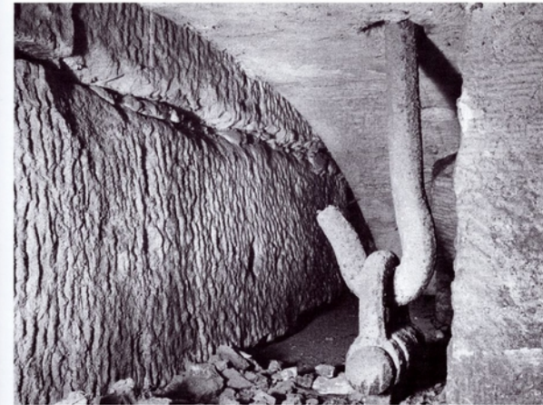
Figure 14.12 West porch, St Paul's Cathedral, London, England (Courtesy: Feilden & Mawson)
